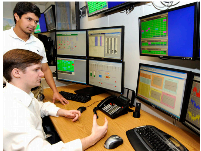
At FPL's Performance and Diagnostic Centers, the company uses smart grid technology to predict and prevent power outages.
